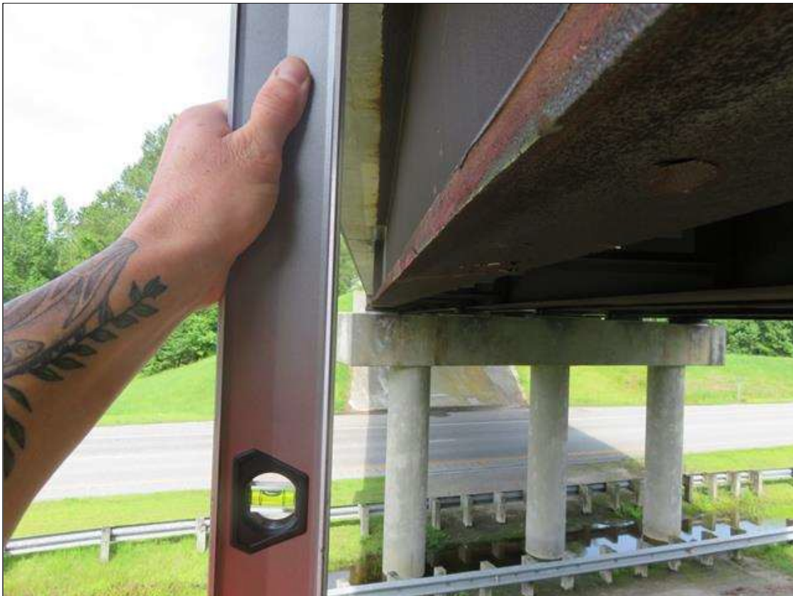
Span 2 Beam 1: BEAM 1 IN SPAN 2 IS BOWED 4" OUT OF PLUM TOWARDS THE WEST @ POINT OF IMPACT FOR OVER HALF THE LENGTH OF BEAM.
