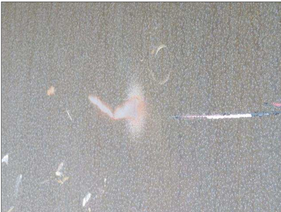
Span 2 Beam 1: 3" DIAMETER X 1/4" DEEP INDENTATION IN BEAM 1 SPAN 2 WEB 17" FROM TOP FLANGE AND LOCATED OVER RIGHT WEST BOUND THRU LANE.
