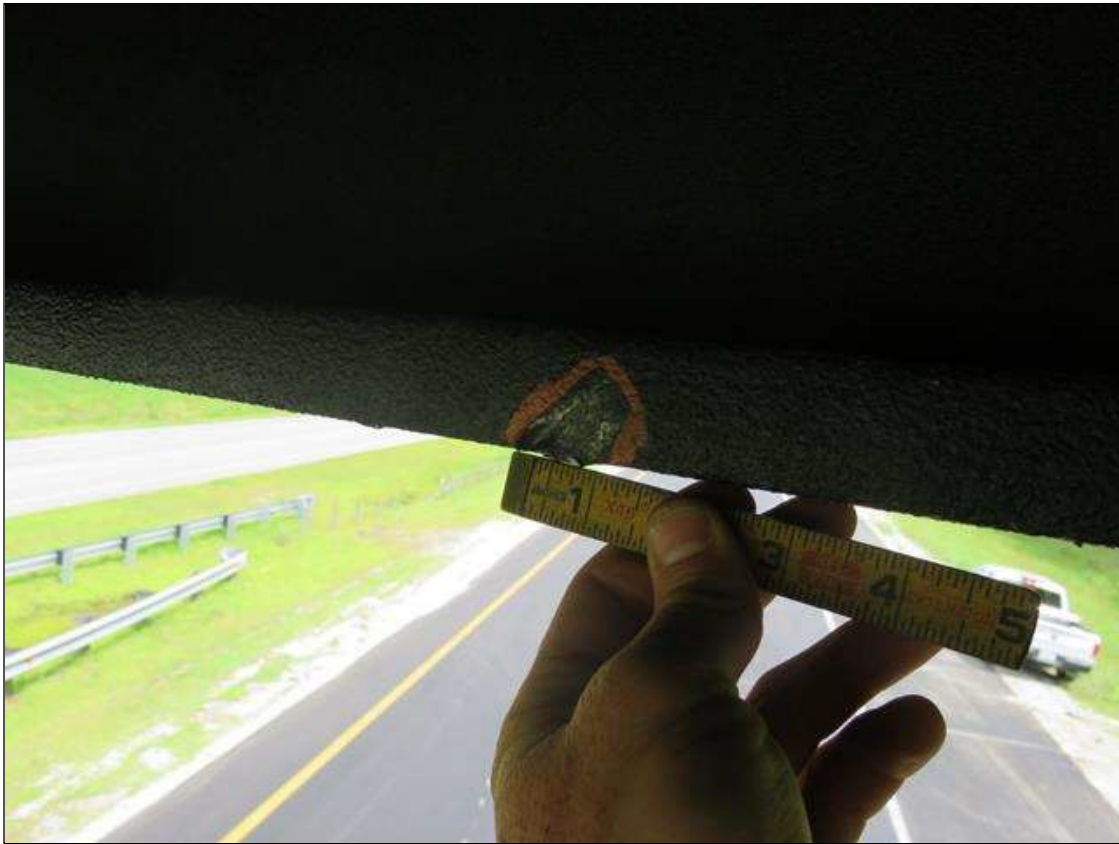
Span 2 Beam 4: 1" WIDE X 1/8" DEEP GOUGE IN BOTTOM FLANGE OF BEAM 4 IN SPAN 2.
