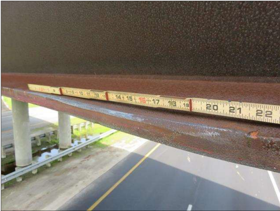
Span 2 Beam 1: BEAM 1 IN SPAN 2 HAS A 21" LONG X 1/16" DEEP GOUGE IN BOTTOM FLANGE & IS LOCATED OVER RIGHT WEST BOUND THRU LANE.
