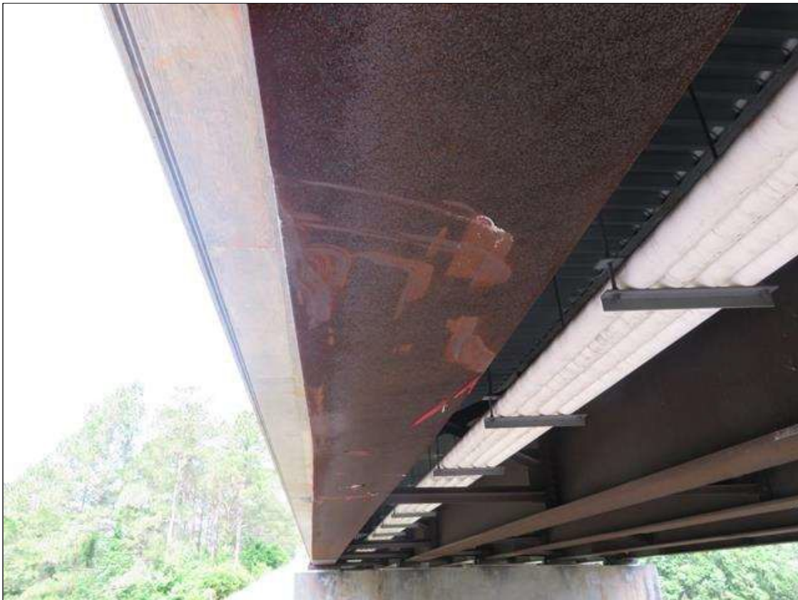
THERE ARE SCRAPE MARKS TO BOTTOM FLANGE OF BEAM 1 IN SPAN 2 FOR AN AREA OF 12 FT LONG.
