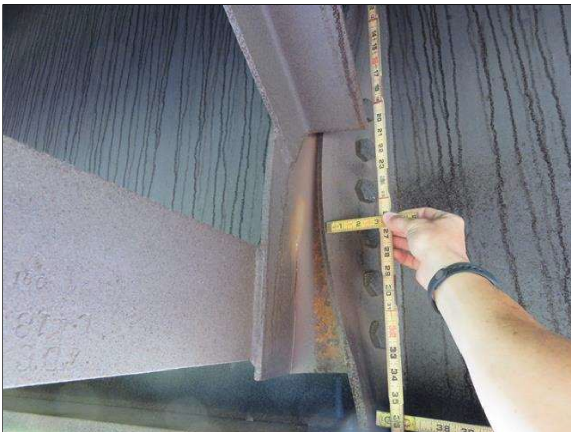
Span 2 Beam 1: INTERMEDIATE DIAPHRAGM 3 IN SPAN 2 BAY 1 CONNECTED TO BEAM 1 HAS AN 8" VERTICAL CRACK AT BOTTOM OF CONNECTION.
