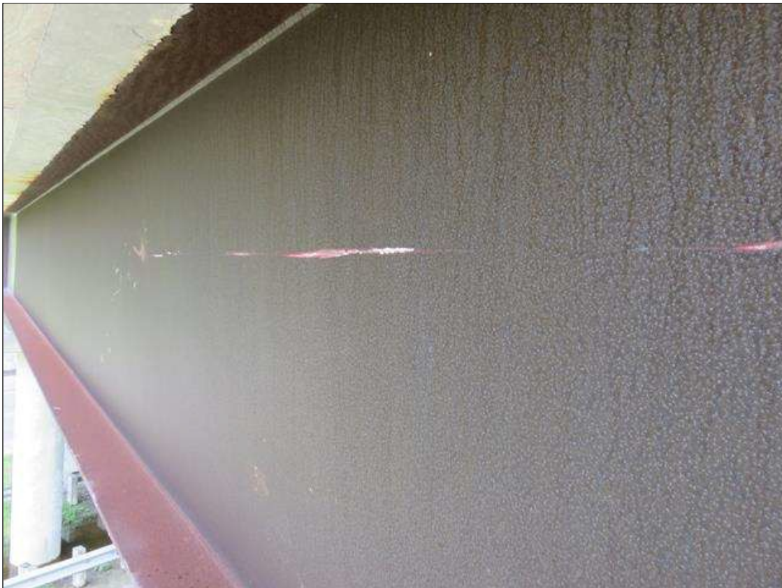
SCRAPE MARKS AND PAINT SMEAR TO WEB OF BEAM 1 IN SPAN 2.
