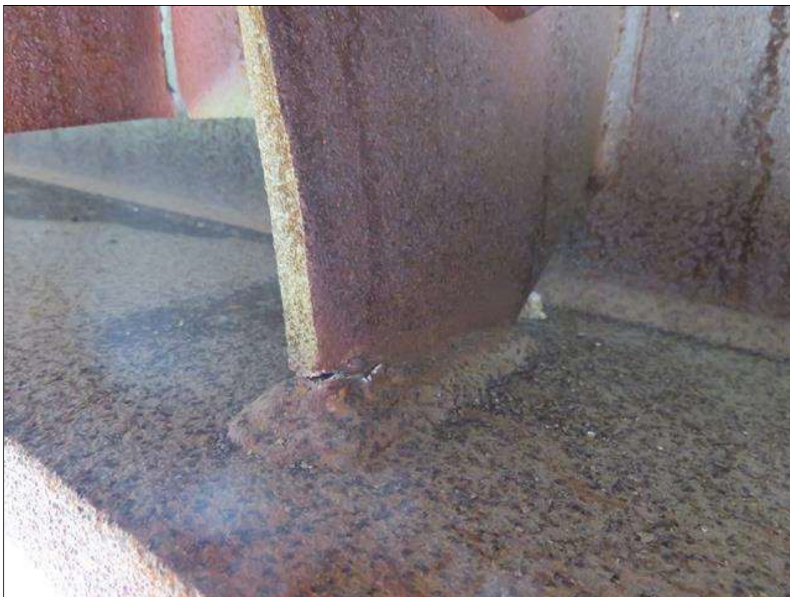
Span 2 Beam 1: 2" LONG CRACK IN WELD TO BOTTOM FLANGE VERTICAL STIFFENER TO INTERMEDIATE DIAPHRAGM 2 IN SPAN 2. OVER LEFT WEST BOUND THRU LANE.
