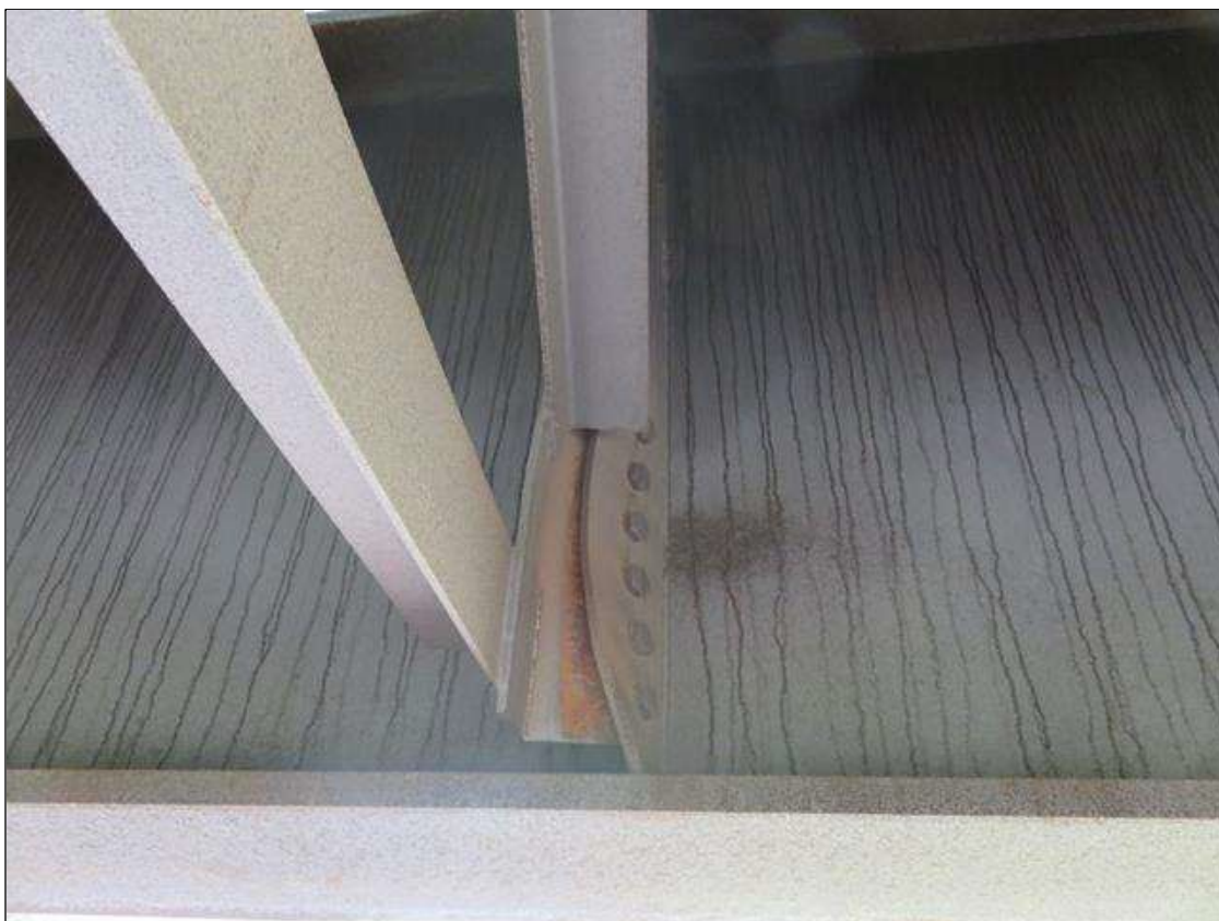
ZOOMED OUT VIEW OF INTERMEDIATE DIAPHRAGM 2 IN SPAN 2 BAY 1.
