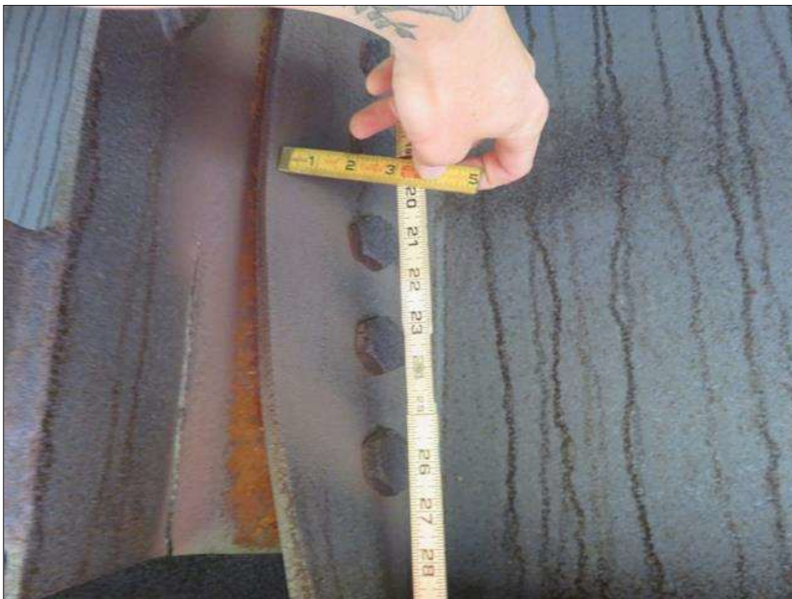
Span 2 Beam 1: 7 1/2" VERTICAL CRACK IN INTERMEDIATE DIAPHRAGM 2 SPAN 2 BAY 1 CONNECTION TO BEAM 1.
