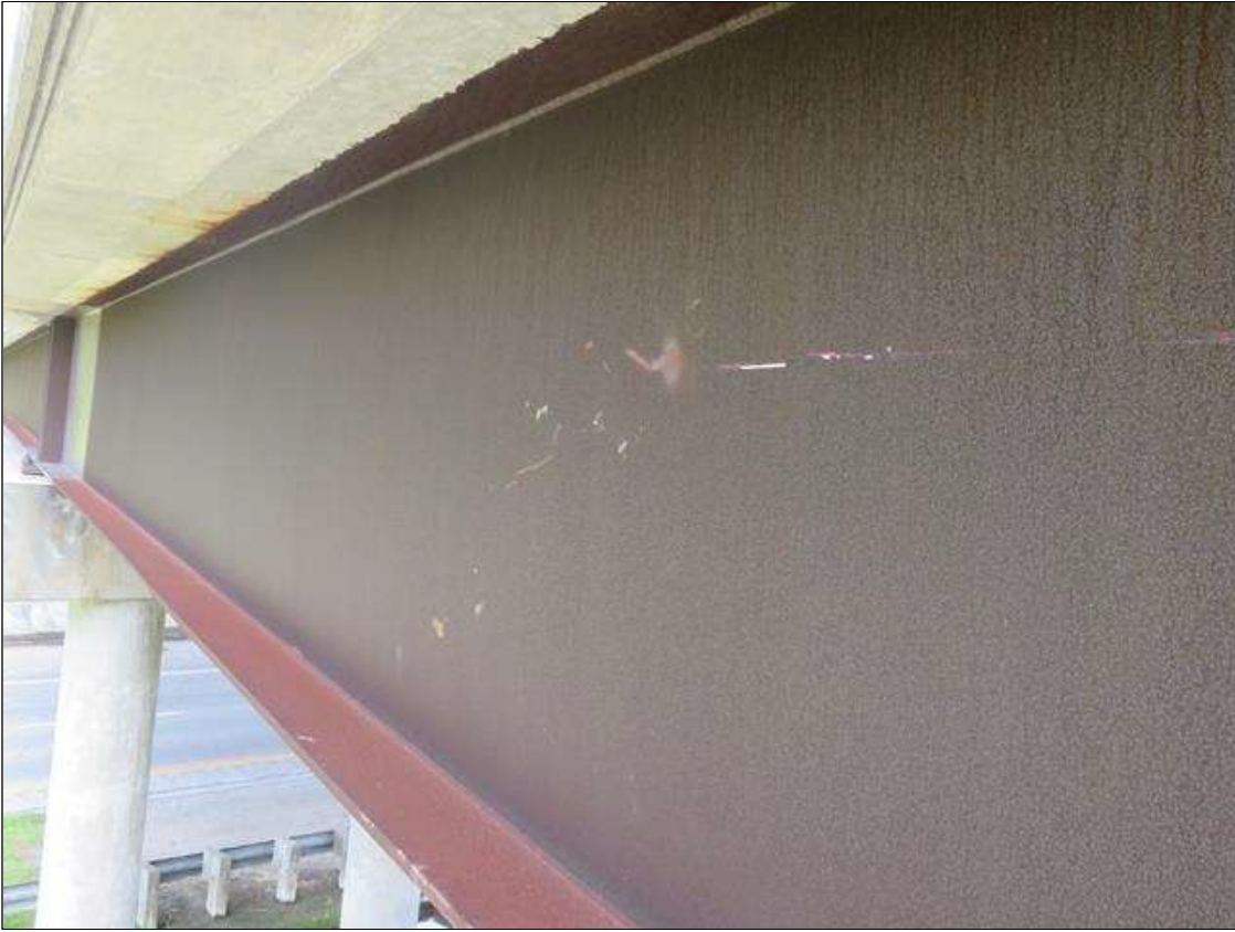
ZOOMED OUT VIEW OF 3" DIAMETER X 1/4" DEEP INDENTATION IN BEAM 1 SPAN 2 WEB. LOCATED OVER RIGHT WEST BOUND THRU LANE.
