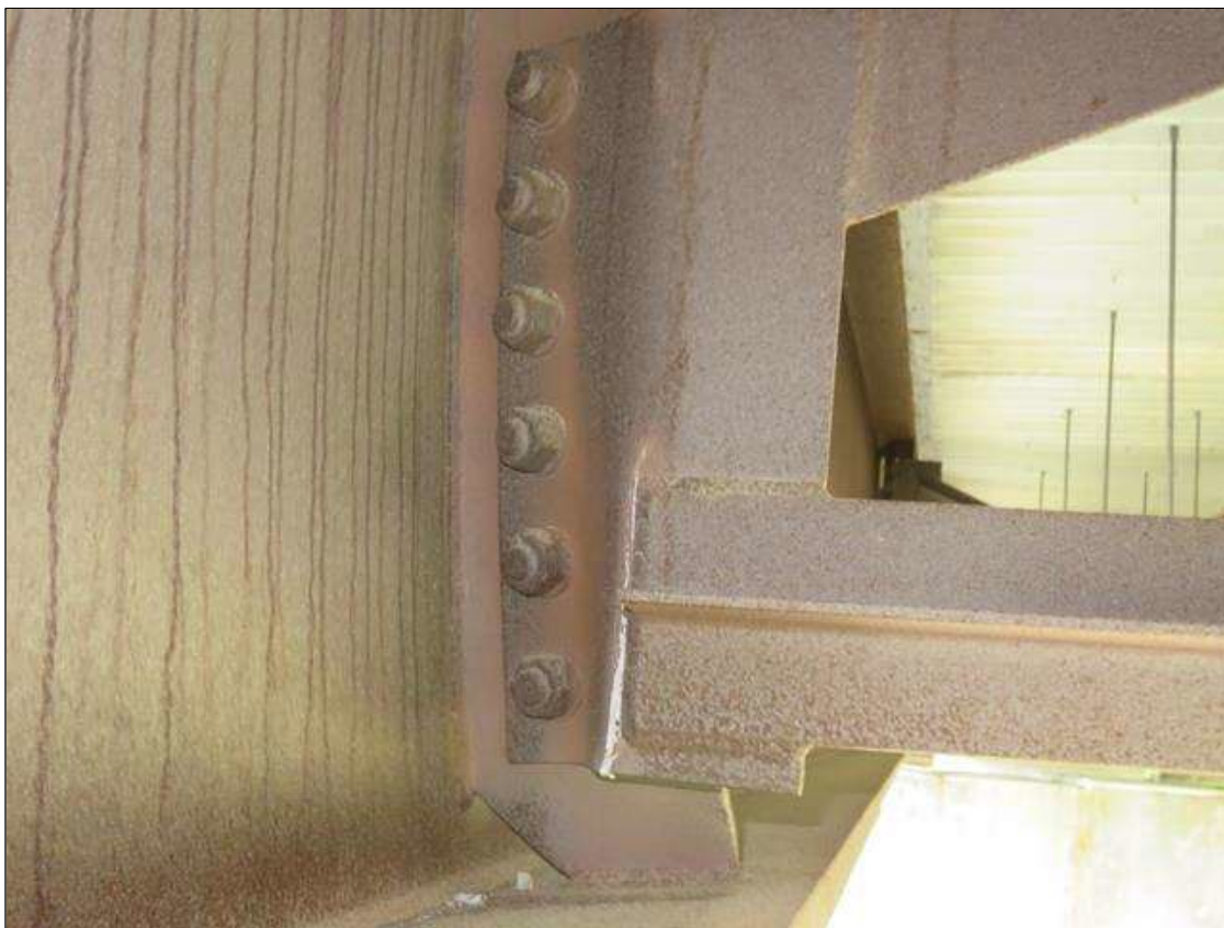
DIFFERENT VIEW OF 7 1/2" VERTICAL CRACK TO INTERMEDIATE DIAPHRAGM 2 IN BAY 1 SPAN 2.
