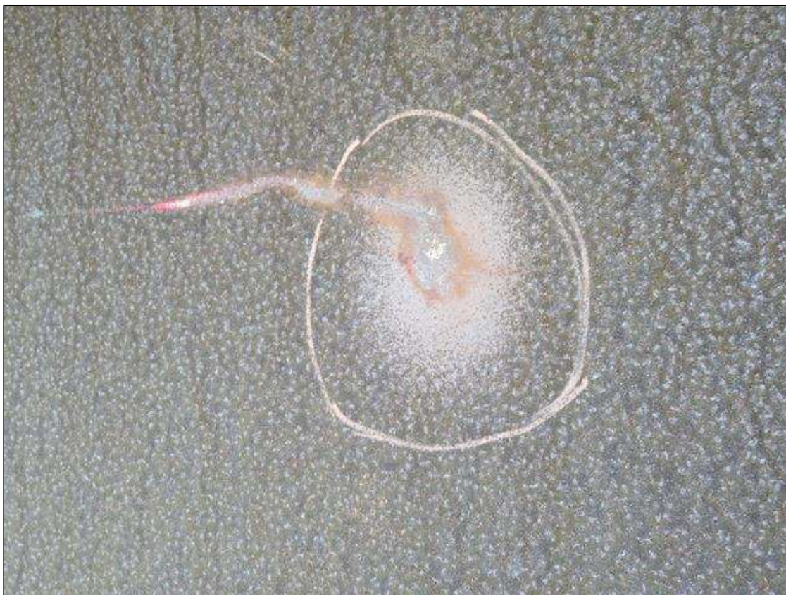
ZOOMED OUT VIEW OF 4" DIAMETER X 3/4" DEEP INDENTATION IN BEAM 1 WEB IN SPAN 2.
