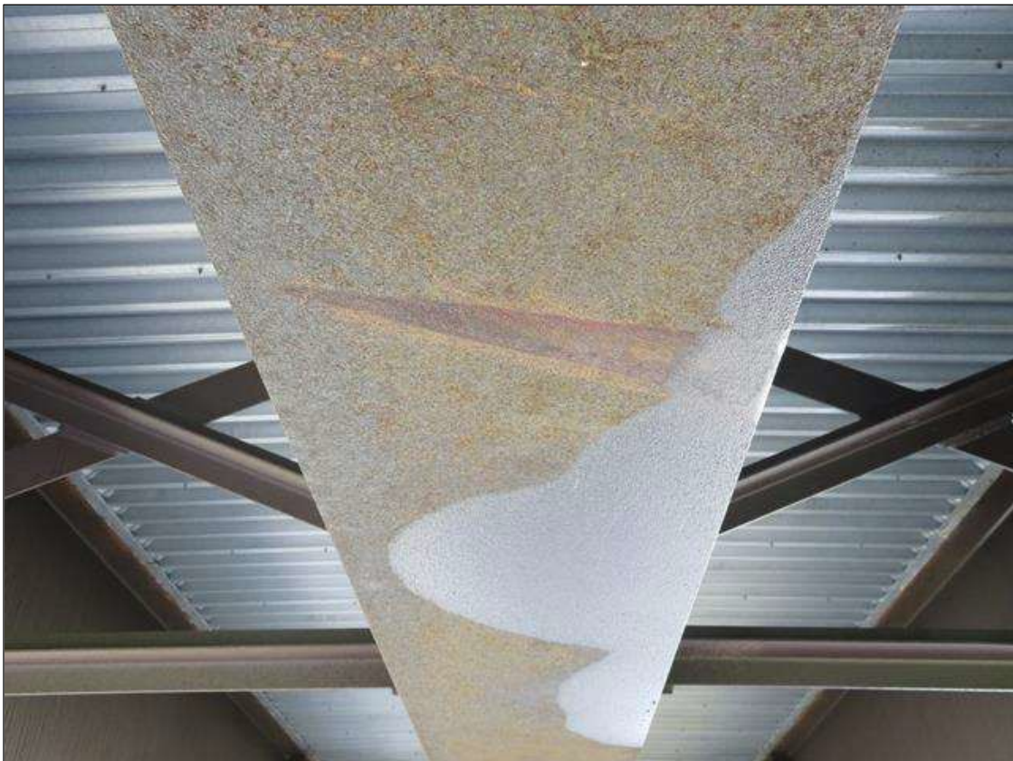
SCRAPE MARK TO BEAM 3 IN SPAN 2 BOTTOM FLANGE.
