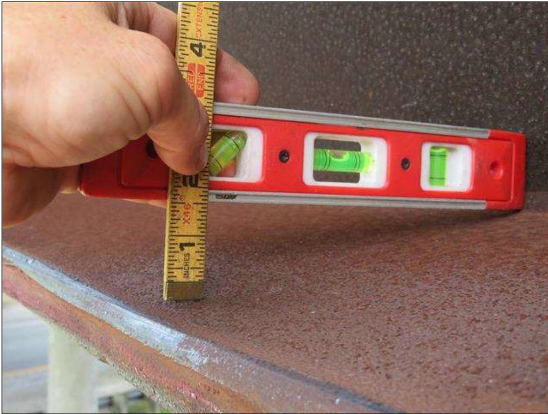
Span 2 Beam 1: BOTTOM FLANGE OF BEAM 1 IN SPAN 2 IS BOWED DOWNWARDS 1 1/2" FOR OVER HALF THE LENGTH OF BEAM AT POINT OF IMPACT
